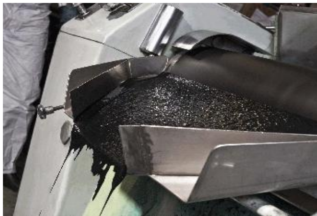
Milling devices in use.
